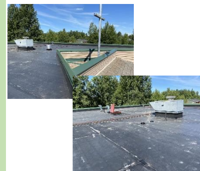
the finished roof
