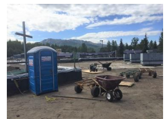
view from the rooftop during construction
